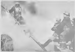
Well protected by fog spray, Marines replace broken bolt in overhead leaking flange.
